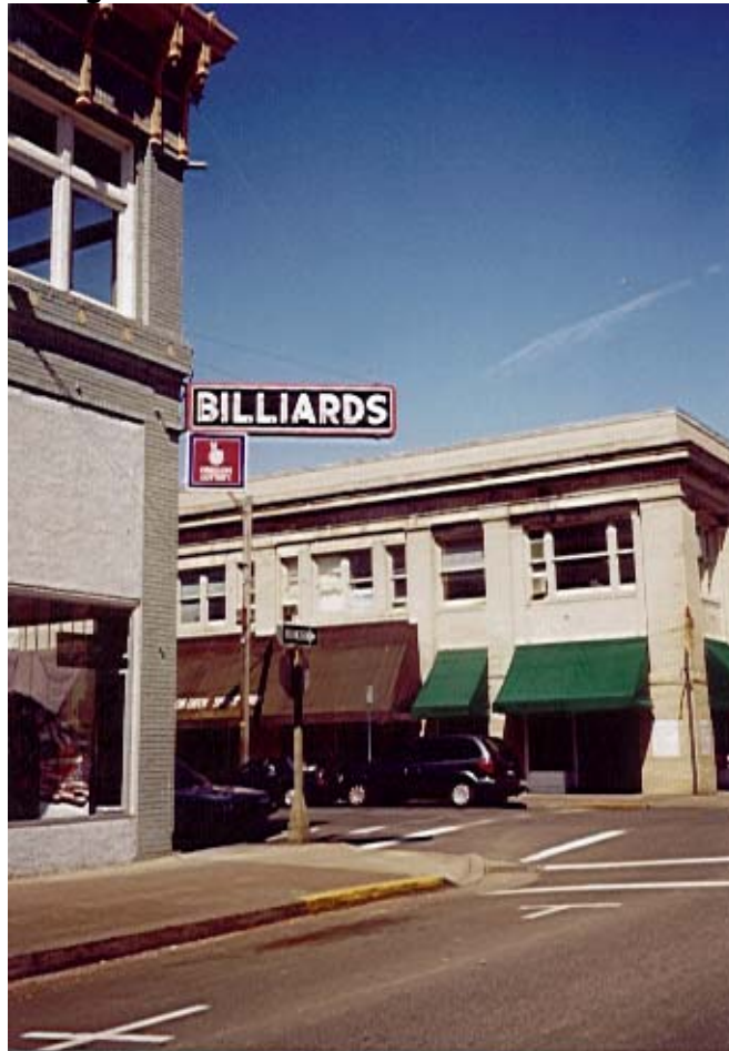
Figure 49 Historic Building at Broadalbin and 2 nd Ave SW, Downtown Albany
