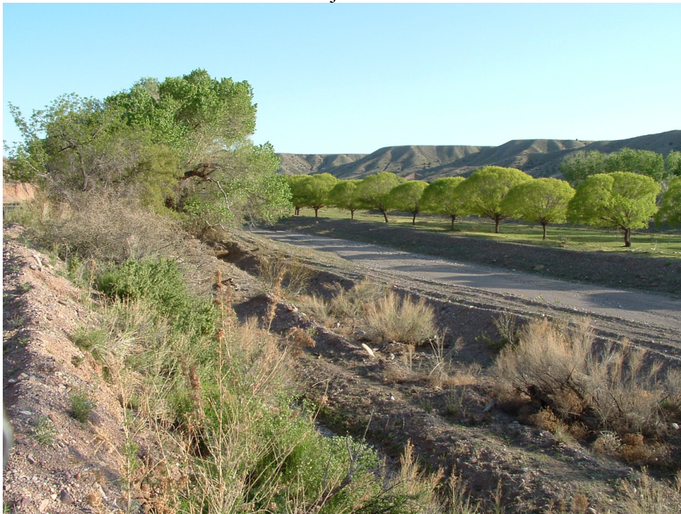
Figure 5.5: Flood Control Project South of Placitas
