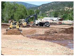
Scott Condon/The Aspen Times | Heavy equipment is working at the former Pan and Fork Mobile Home Park site in Basalt to raise the elevation out of the flood plain closes to Two Rivers Road.
