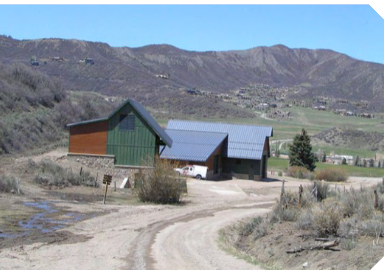
The GIS substation was placed on the site that the citizens chose. The 25 kv distribution lines feed from substation. The public hiking trail incorporated into the site plan is in the foreground.
